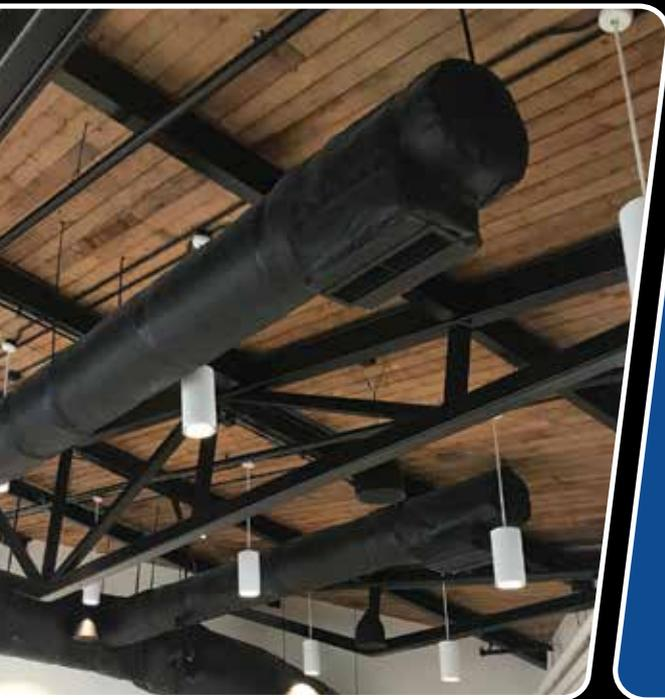
JM's Microlite® **BLACK PSK** Fiberglass Duct Wrap is ideal for applications that call for a sleek, sophisticated look. Now, you can insulate with aesthetics in mind without sacrificing any performance characteristics.
